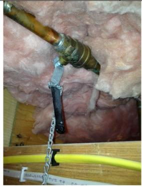
Move handle perpendicular to pipe to close
